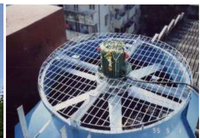
Round-shaped cooling towers. Cooling towers come in various shapes, sizes, material including fiberglass, and configurations.
