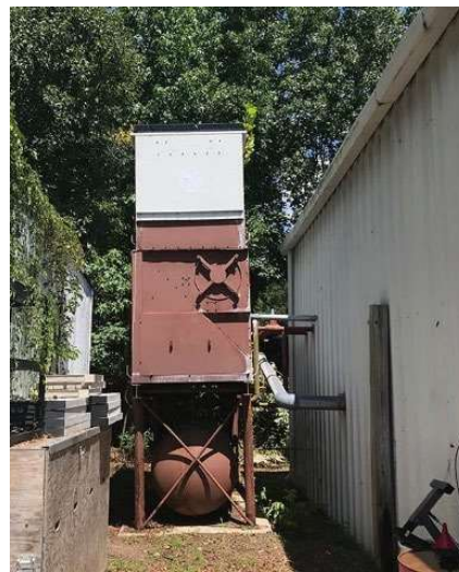
An elevated fully enclosed cooling tower basin with access hatch and a side fan that is not visible.
