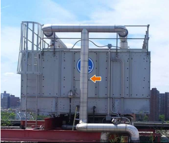
A large cooling tower with easily visible water pipes (highlighted with an arrow).
