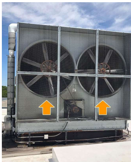
A cooling tower with front facing fans (highlighted with arrows).
