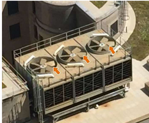
A cooling tower with easily visible fan blades (highlighted with arrows).
